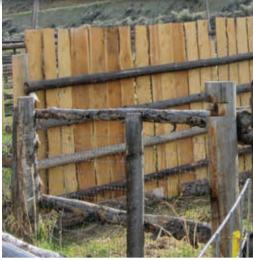
Windbreaks are often made with boards placed vertically, leaving spaces between them. The target porosity is from 20% open and 80% solid to 65% or 70% solid.
