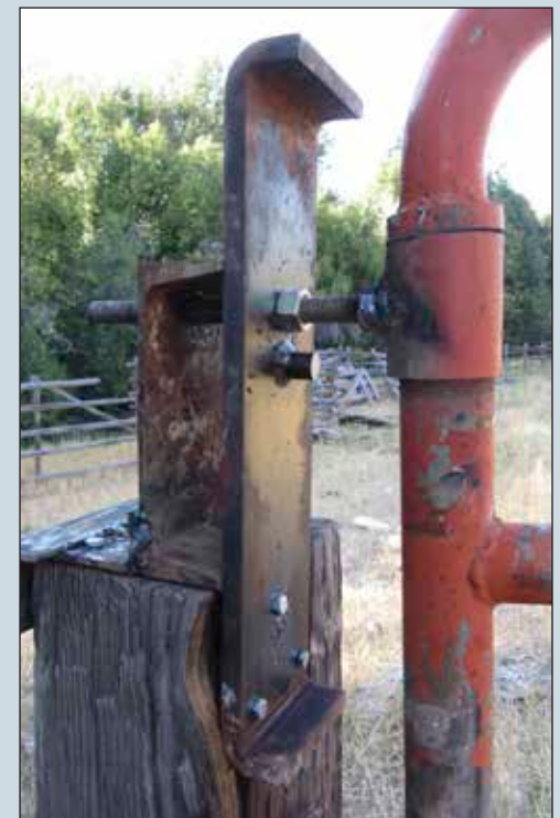
Fig. 10: Post extension to support gate
