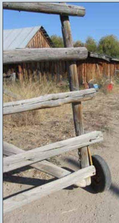
Fig. 9: Example of wheel on gate
