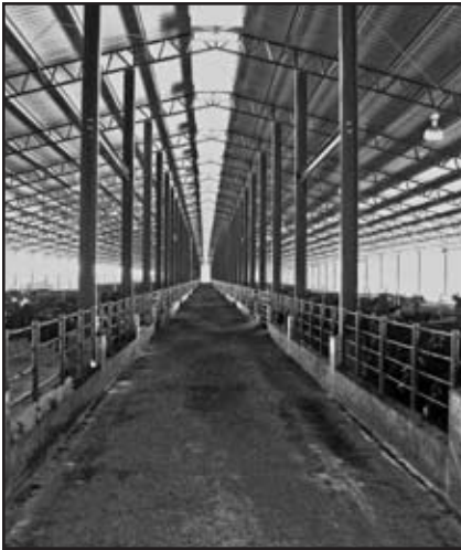
Circle A Feeders' 5,000-head yard is one of the largest building-enclosed feedlots in the U.S. The climate in central Missouri and the production of black cattle were deciding factors in covering the yard.
