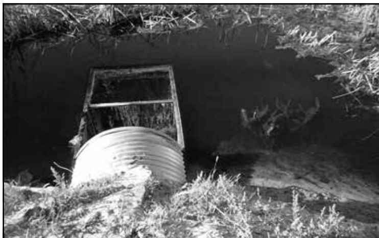
At the site of a vehicle crossing, a weir was installed on one of the Cedar River's tributary creeks. Designed to enhance water flow and stabilize creek banks, as well as the crossing, weir construction is an example of Pelster Ranch conservation projects completed in cooperation with the Natural Resources Conservation Service and other agencies.
