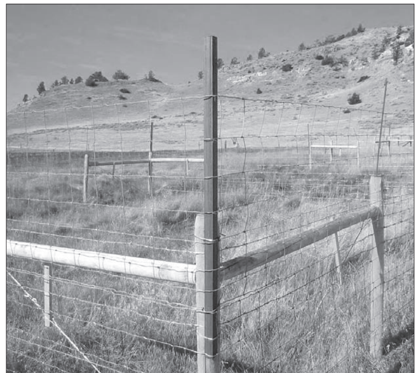
An MSU study indicates a 6-ft. woven-wire fence is the best line of defense against hungry deer.
