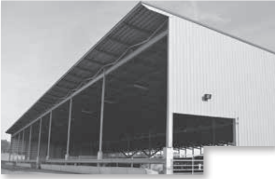
Left: While there are less-expensive options, they decided on a monoslope building because of greater building longevity. Monoslope barns provide better natural ventilation, sunlight, shade and shelter from the elements, like Indiana's average 40 inches of rainfall.
