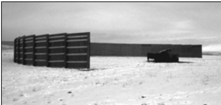
Bob Jairell, retired FS researcher, prefers a solid snowbreak to protect cattle from snow and wind.
